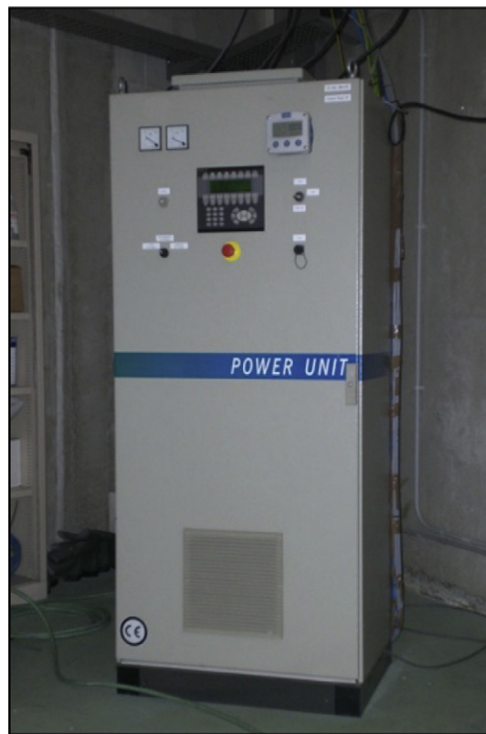
FIGURE 14.16 Commercial power and control unit for the alkaline electrolyzer, model H2 IGEN 300/1/25. (For color version of this figure, the reader is referred to the online version of this book.)
